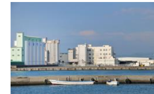
Tokyo factory (Pre-mix production)
